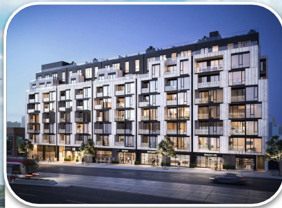
836 St Clair Ave W 8 Storeys 116 Units
